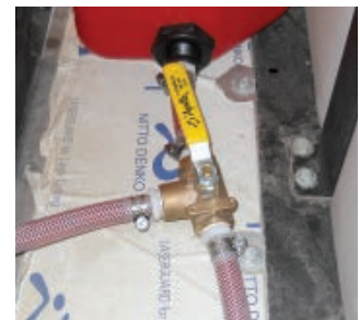
Valve position for water
