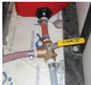
Valve position for antifreeze
